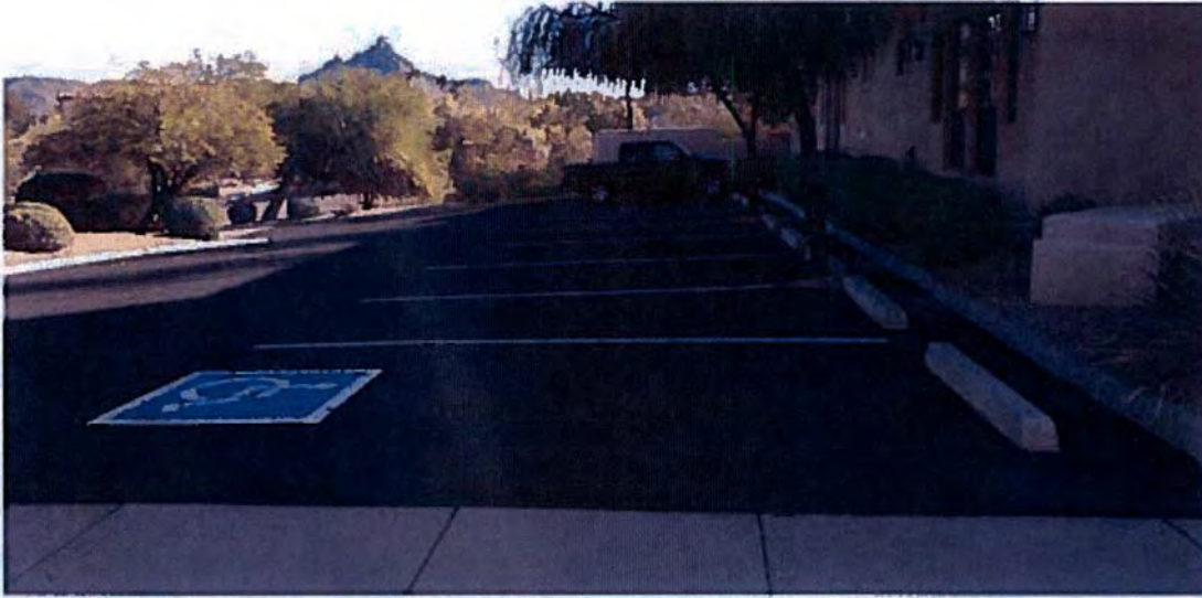
IMAGE #7 at North Side Looking at Existing Parking Area
