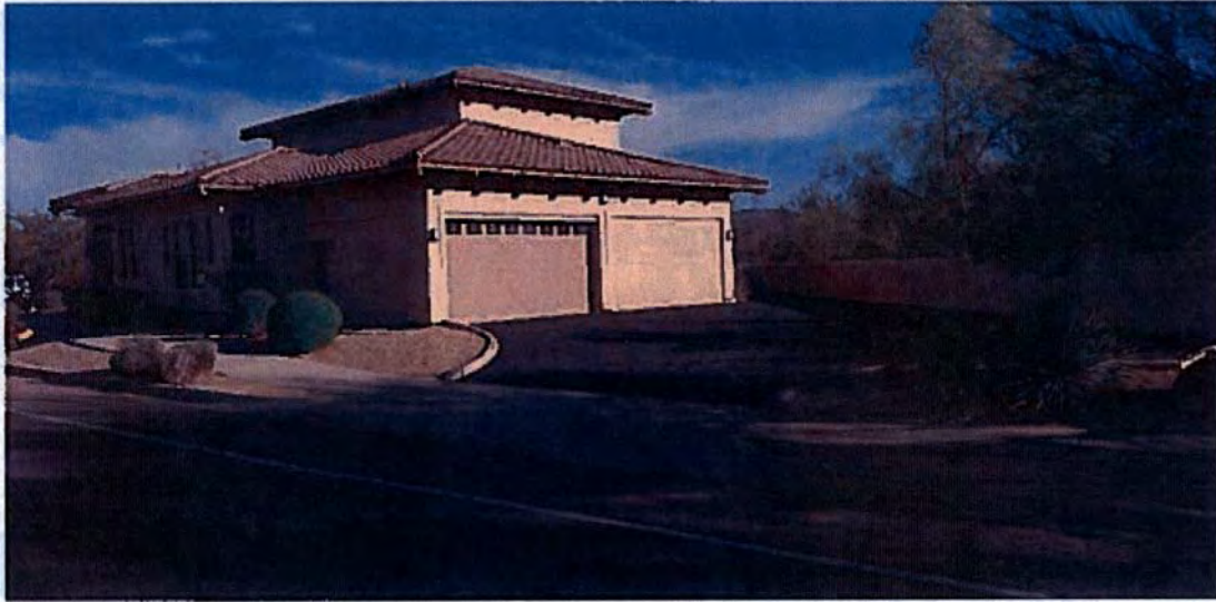
IMAGE #5 at North-West Corner Looking at Existing Driveway
